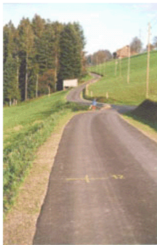
Stabilized, solid after TerraDry treatment
