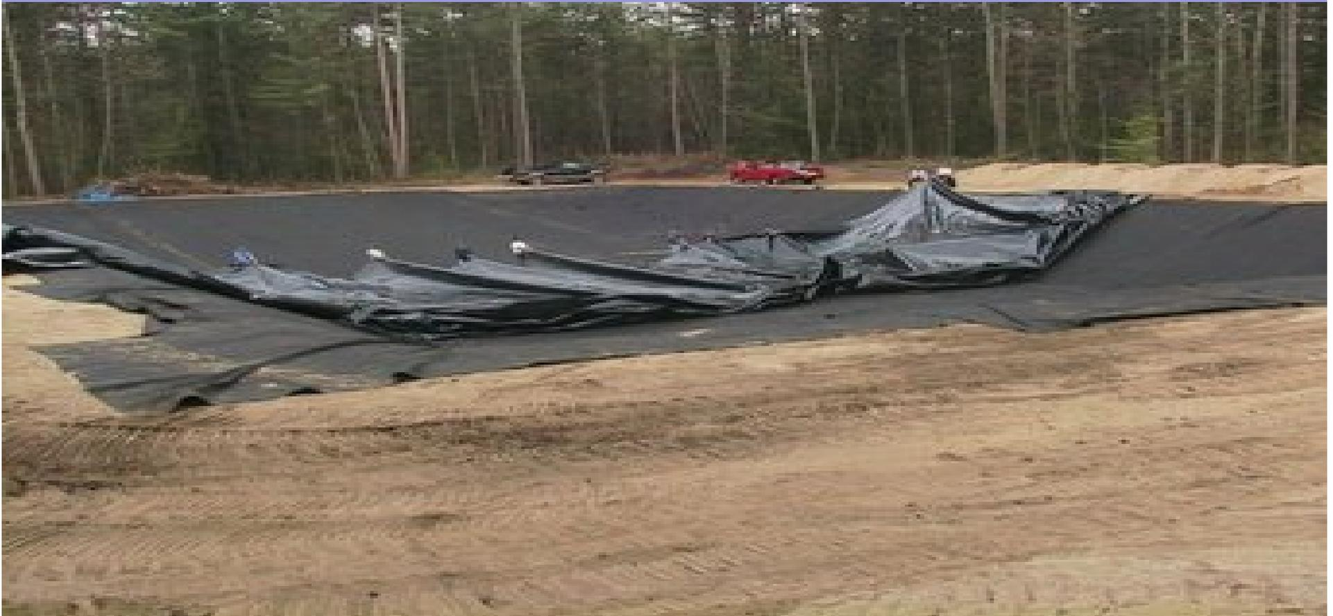
Continue to unfold, pulling to desired location leaving approximately 5% slack for material contraction purposes.
