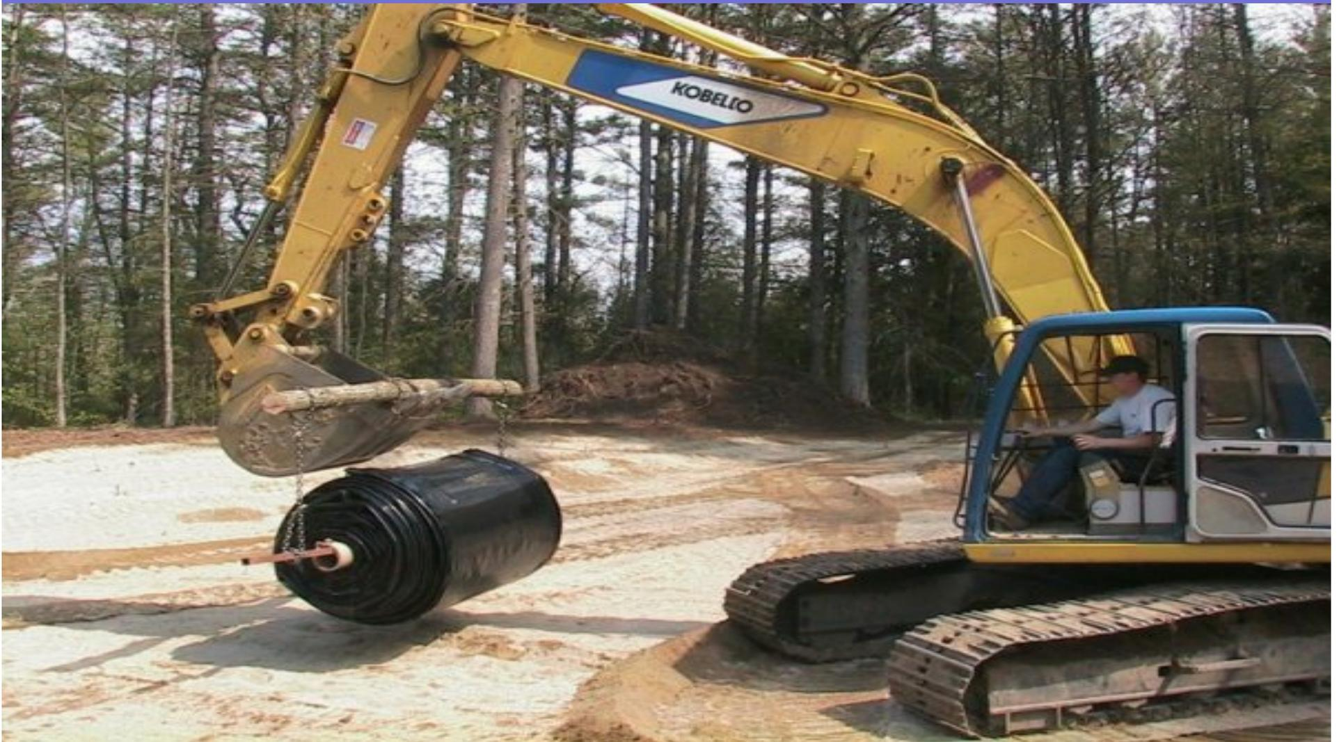
This is the WRONG WAY to hook up the chains. The chain will damage the material during deployment.
