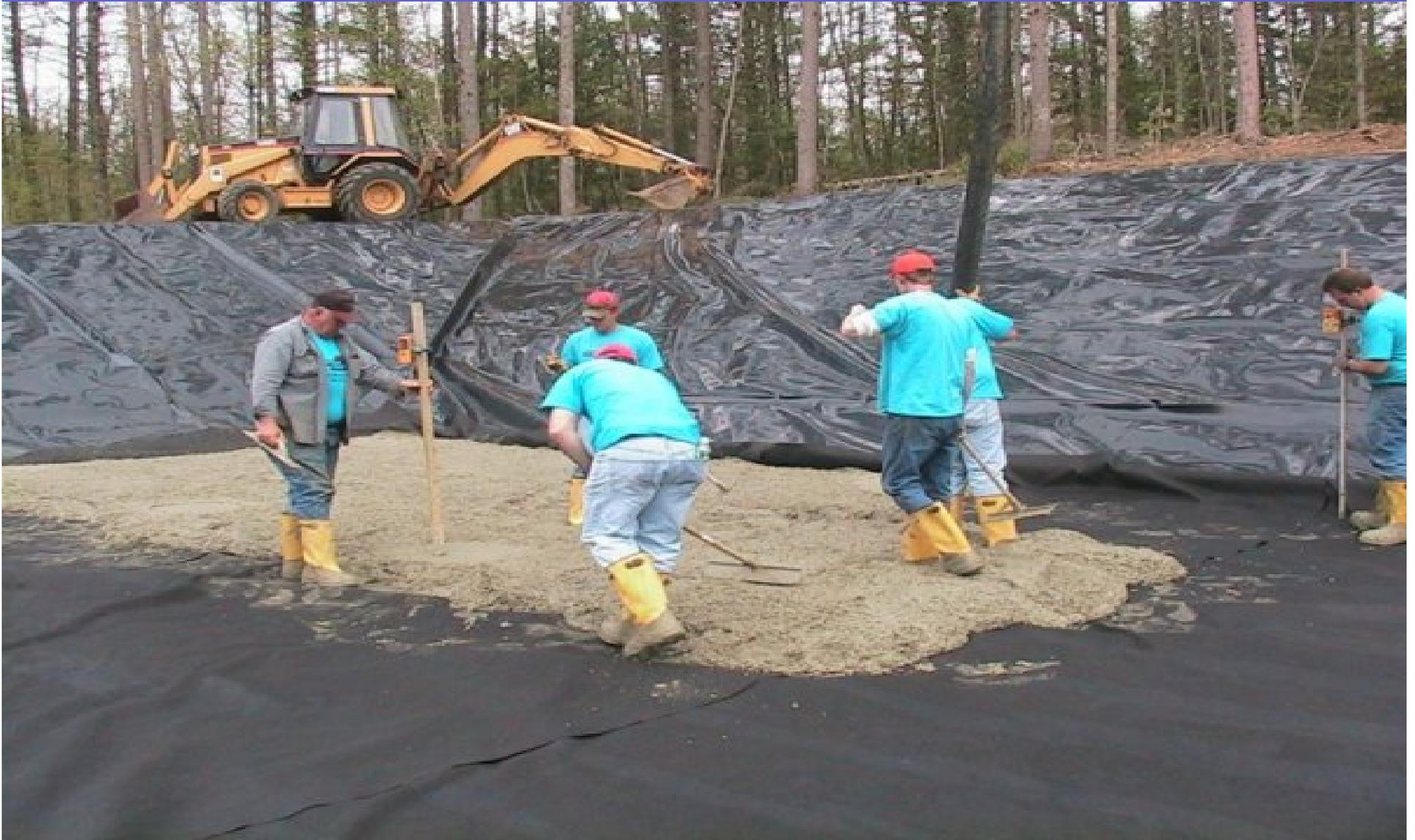
Depending on application, secure around perimeter with appropriate procedure. For example an anchor trench is used below.
