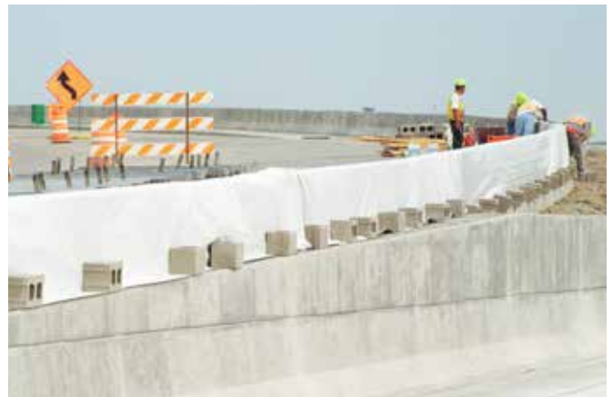
Wet Curing Blanket
