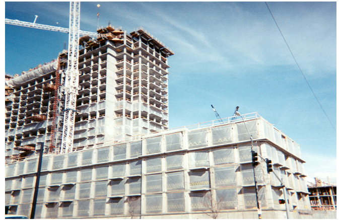
Building Abatement Enclosure
