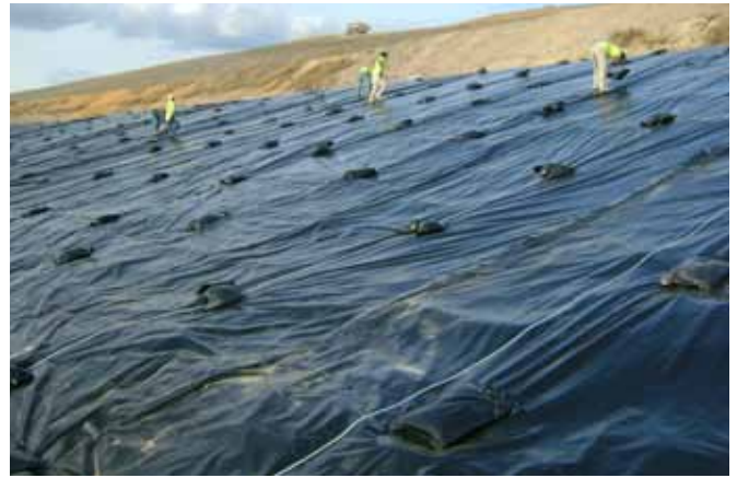
Temporary Rain Shed Cover
