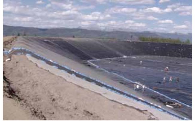
Containment Pond Liner
