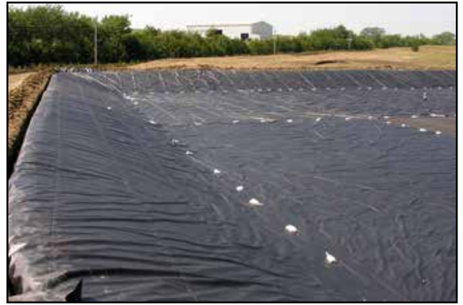
Waste Containment Liner
