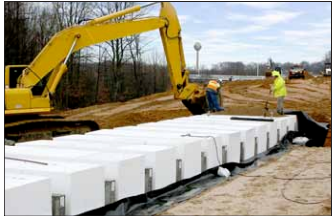
EPS Geofoam Protection
