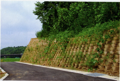
The wall was soon supporting the growth of native grasses, wildflowers, and ferns.
