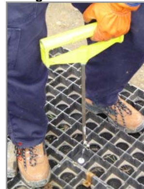
Figure 2 Driving the Anchor Head
