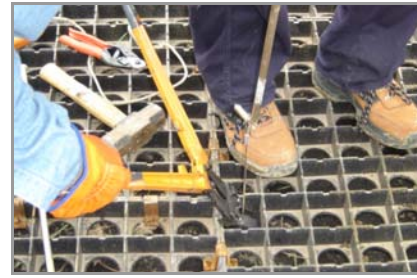
Figure 4 Crimping the Cable Stop
