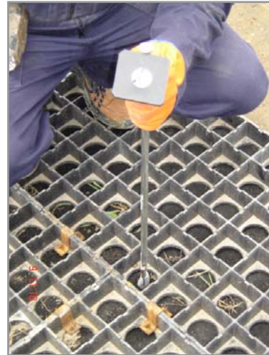
Figure 1: Installing the Earth Anchor
