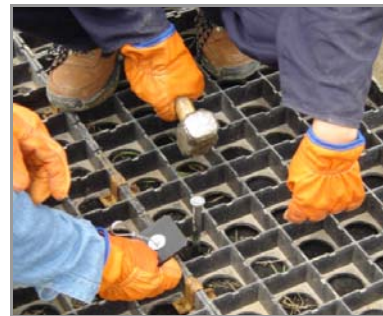
Figure 2 Driving the Anchor Head
