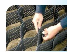
Infill type varies from vegetation to aggregate and hard-armored concrete.
