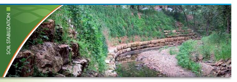
The GEOWEB® Channel Protection System stabilizes and protects channels exposed to erosive conditions of all types and can be designed with appropriate infill types to withstand even the highest velocities.
