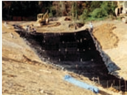
Stabilized Spillway with Geoweb®/TRM Solution
