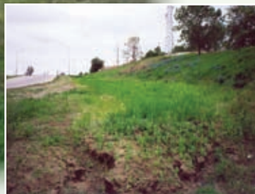
Typical Ditch Erosion Problem
