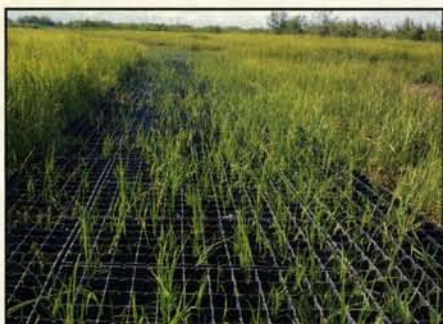
Open grid cell allows for vegetation re-growth.
