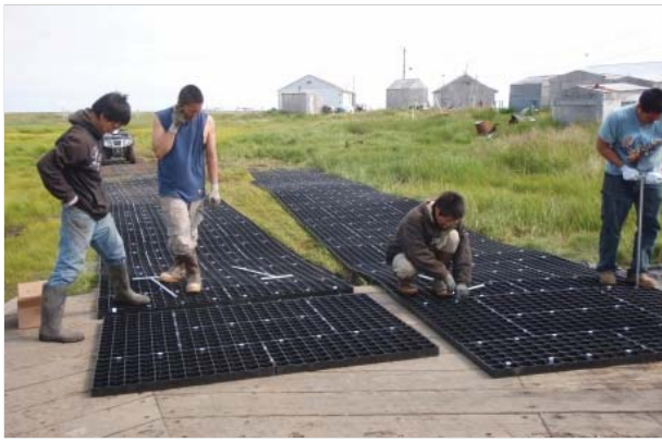
The trailbuilding units formed an interconnected structural mat pavement system. Photo courtesy of the author.
