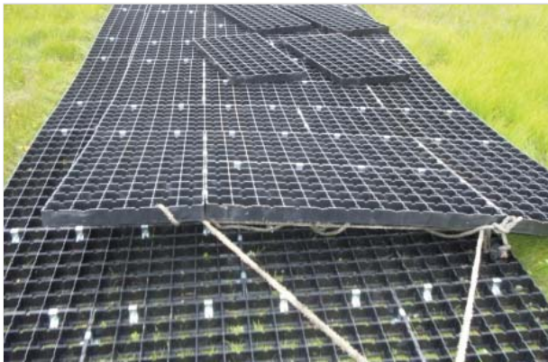
Moving pre-assembled 50-ft mat sections into position with ropes tied to ATVs. Photo courtesy of the author.
