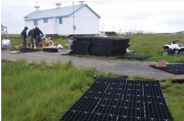
Moving pre-assembled 50-ft mat sections into position with ropes tied to ATVs. Photo courtesy of the author.
