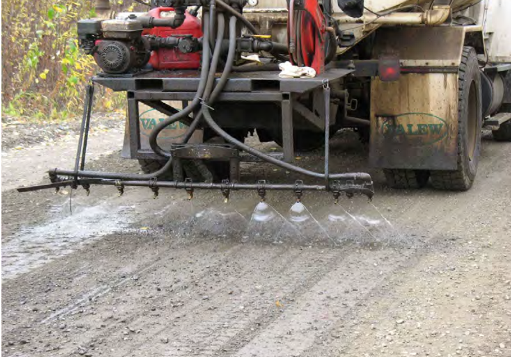
Tanana. Brice, Inc. (airport contractor) Road Work, applying TerraLock in Fall 2007.
