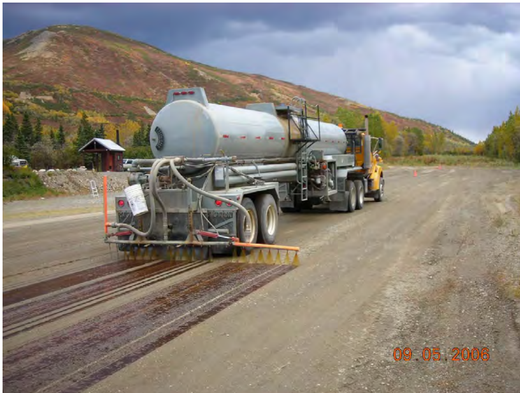
Kantishna airstrip. NPS applying product in 2006.
