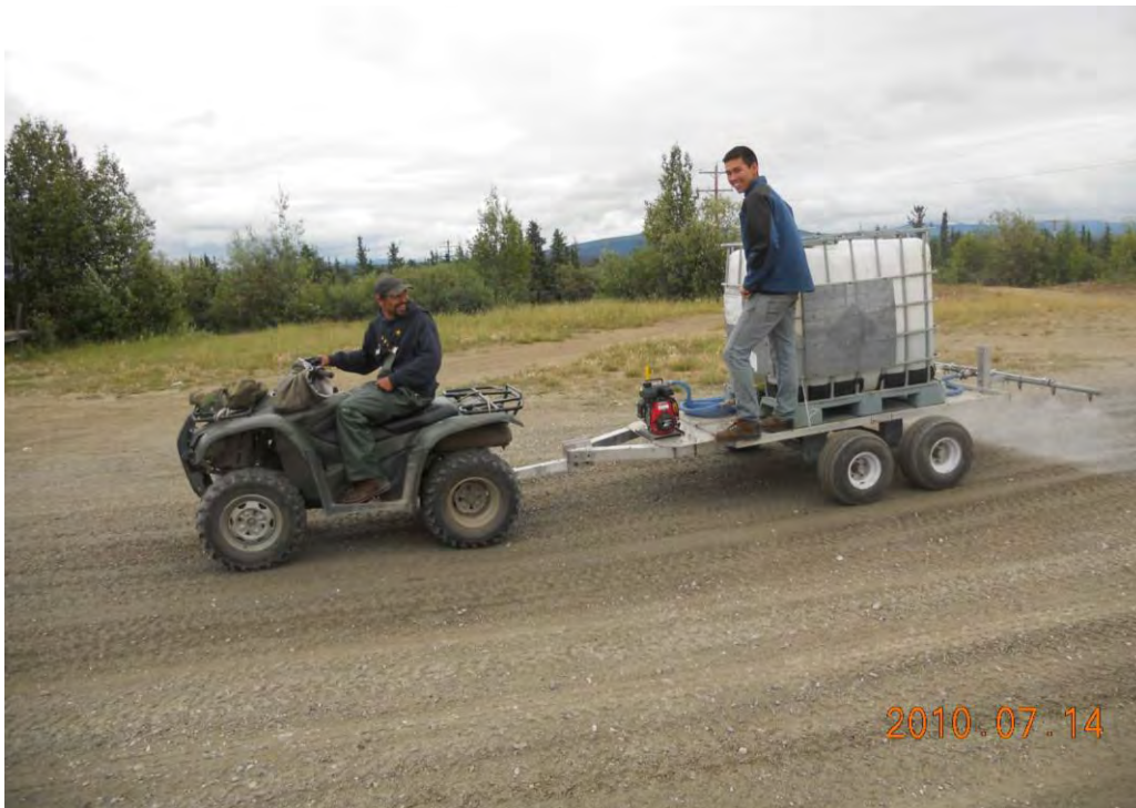
Ambler roadway, "8 Villages Project". "Practice" spraying (water) with Apun sprayer; July 2010
