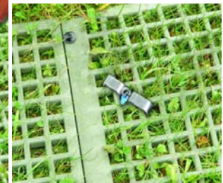
Figure 9. Loop cable back in the Gripple
