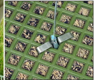
Figure 7. Set Gripple in anchor brace.
