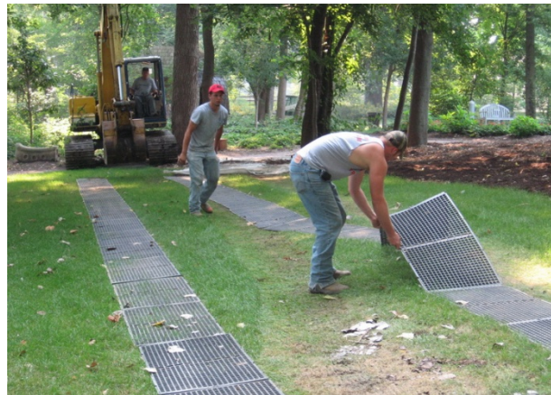
Figure 1. GeoRunner Panel Installation
