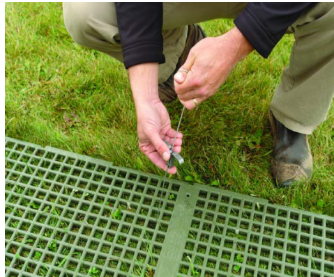
Figure 6. Install Anchor Brace/Gripple
