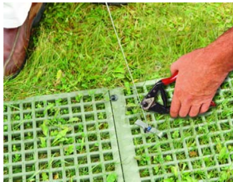
Figure 8. Cut the cable to loop the trailing end
