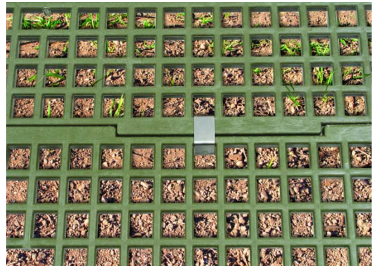
Figure 3. Connect Panels with Side Clips
