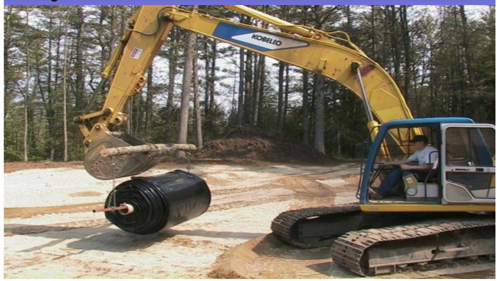
This is the WRONG WAY to hook up the chains. The chain will damage the material during deployment.
