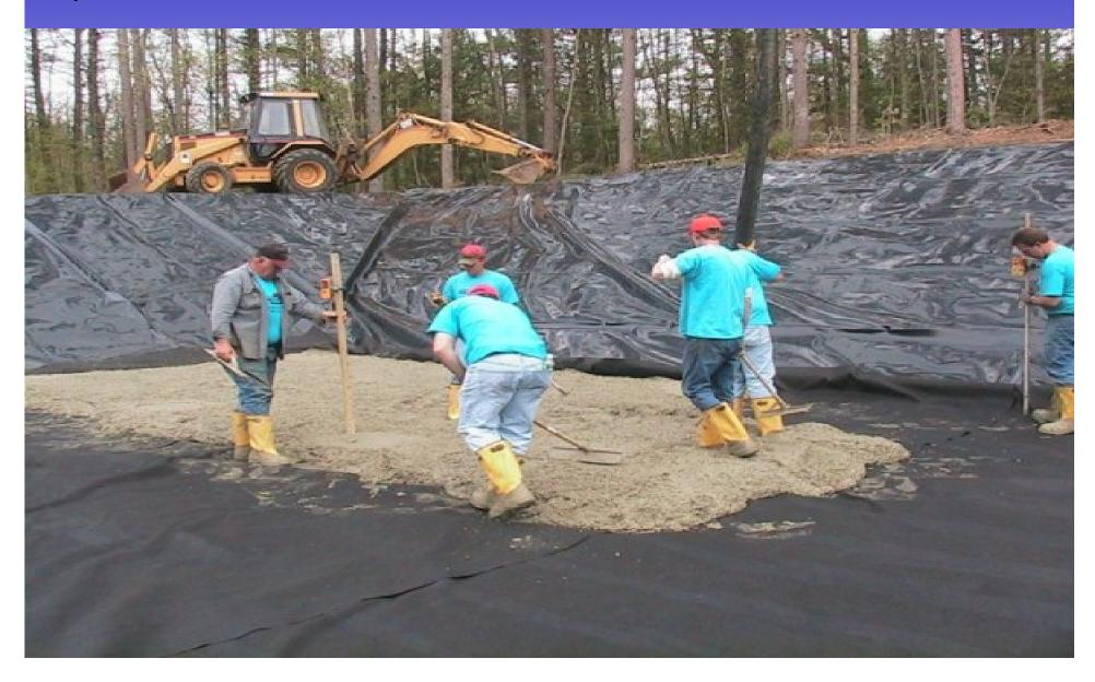
Depending on application, secure around perimeter with appropriate procedure. For example an anchor trench is used below.
