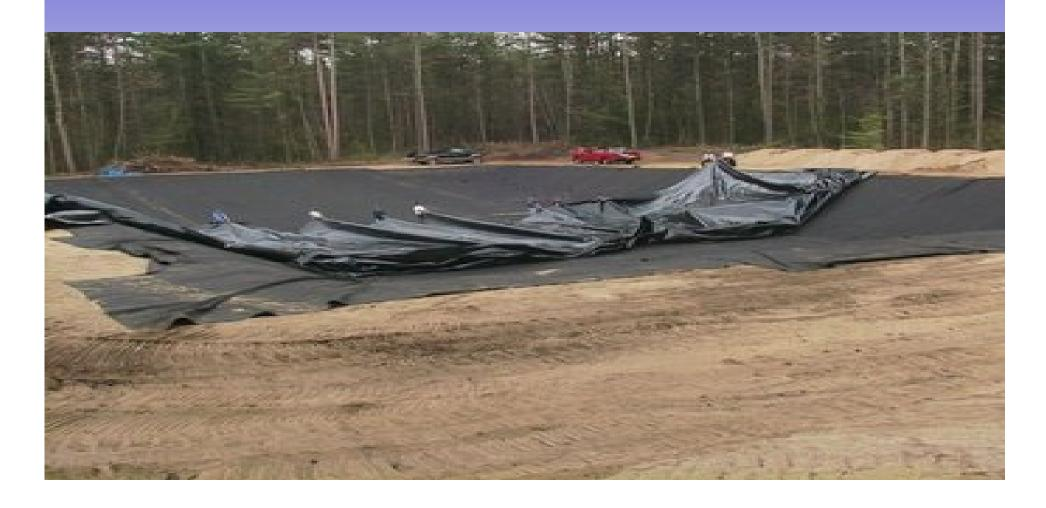
Continue to unfold, pulling to desired location leaving approximately 5% slack for material contraction purposes.
