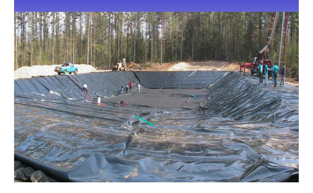
Ballasting the liner: In this case they are using concrete to ballast the liner. A ballast may consist of anything that will hold the liner in place but not harm the liner.
