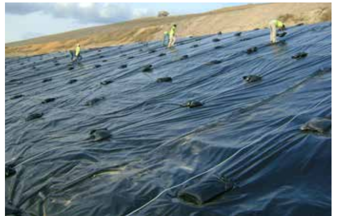
Temporary Rain Shed Cover
