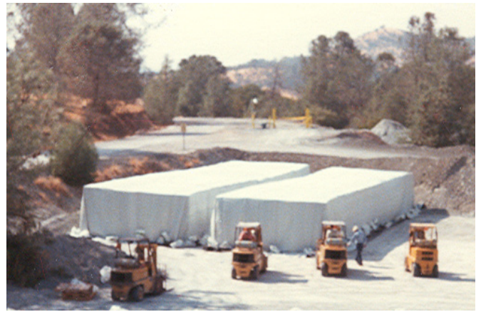
Construction Site Covers
