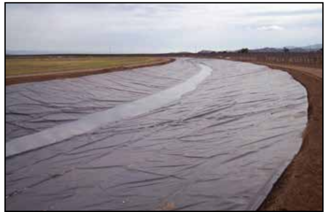
Irrigation Canal Liner
