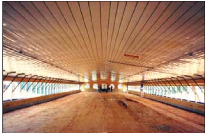
Poultry House Ceiling
