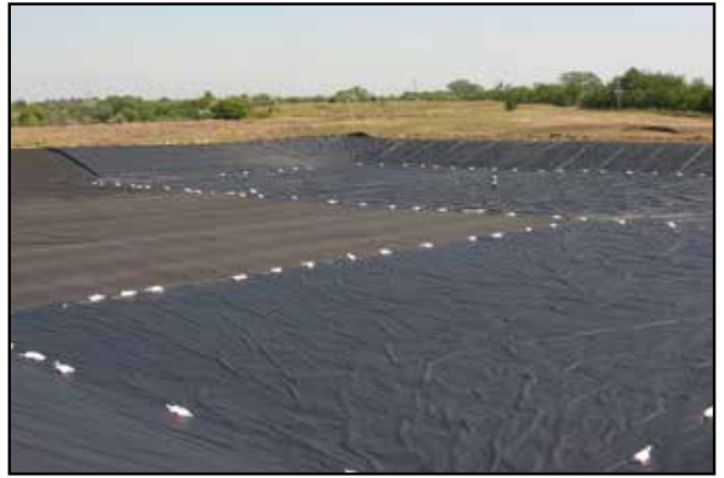
Waste Containment Liner
