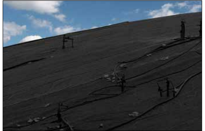
Landfill Odor Control Barrier
