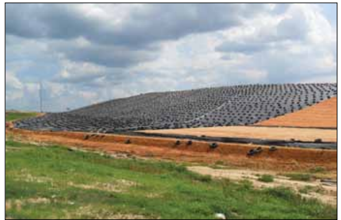
Temporary Landfill Cover
