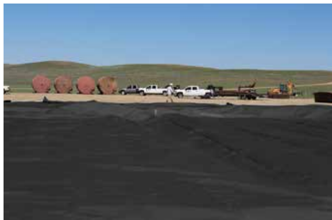
Rig-Site Pad Liner
