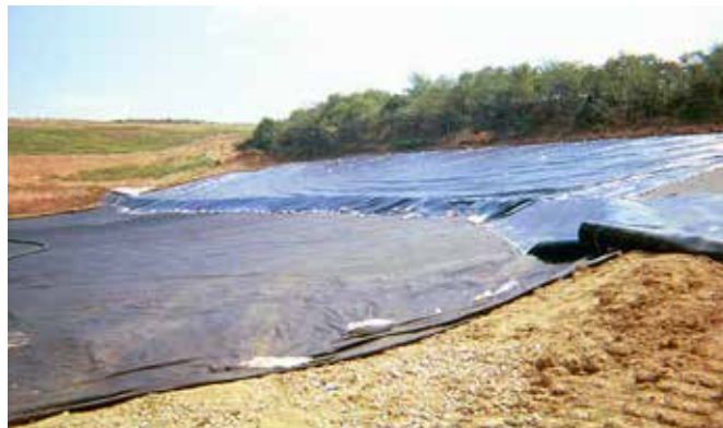
Interim Landfill Cover
