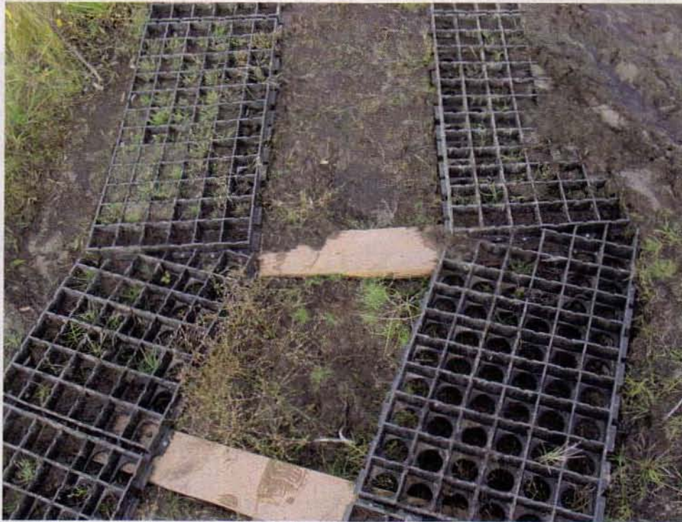
Photo 5. Detail of an orner joint. This technique allows for a quick overlap or miter joint supported by a standard cross tie. A chainsaw is used to make the cut.
