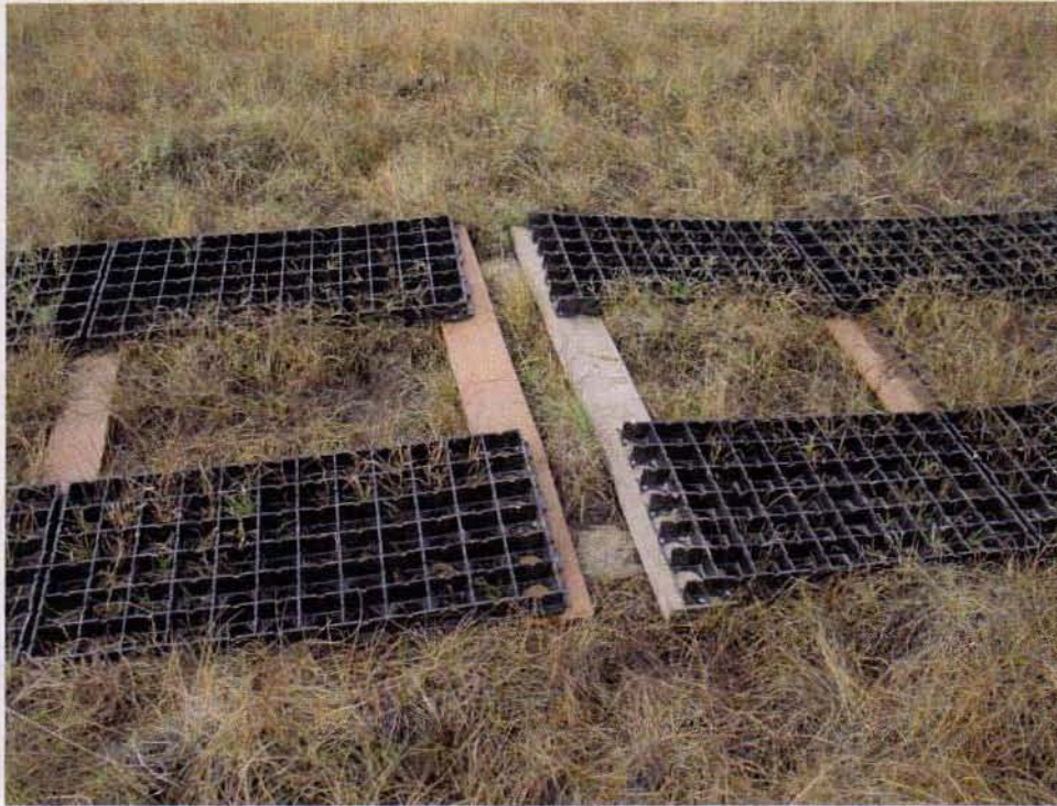
Photo 6. Detail of a thermal expansion joint. These are required every 60-80 feet along the installation to provide for panel shrinkage and swelling. Note use of 2X6 skid platse under panel-end cross ties. The gap (approximately 6 inches) between the panels is easily crossed by ATVs.
