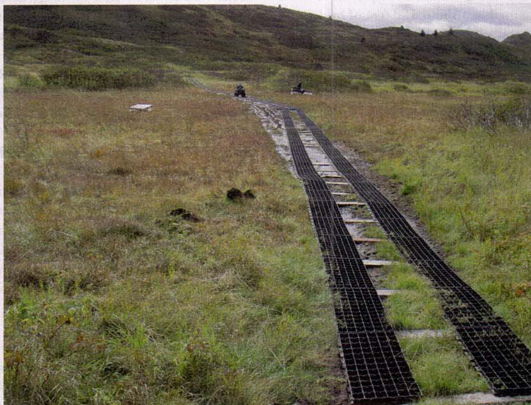
Photo 1. Typical layout of GeoBlock "Geotrack" configuration using 2 inch thick GeoBlock panels and 5 foot wide pressure treated 2X6s as cross ties. This section is installed along a new alignment of the trail. The panels are attached to the cross ties with 1 5/8" long deck screws. Utilizing this approach, only two GeoBlock panels are required for every meter of trail verses three panels for the more common full panel width configuration. This method promises to be a highly effective trail hardening method across a wide range of application sites in Alaska.
