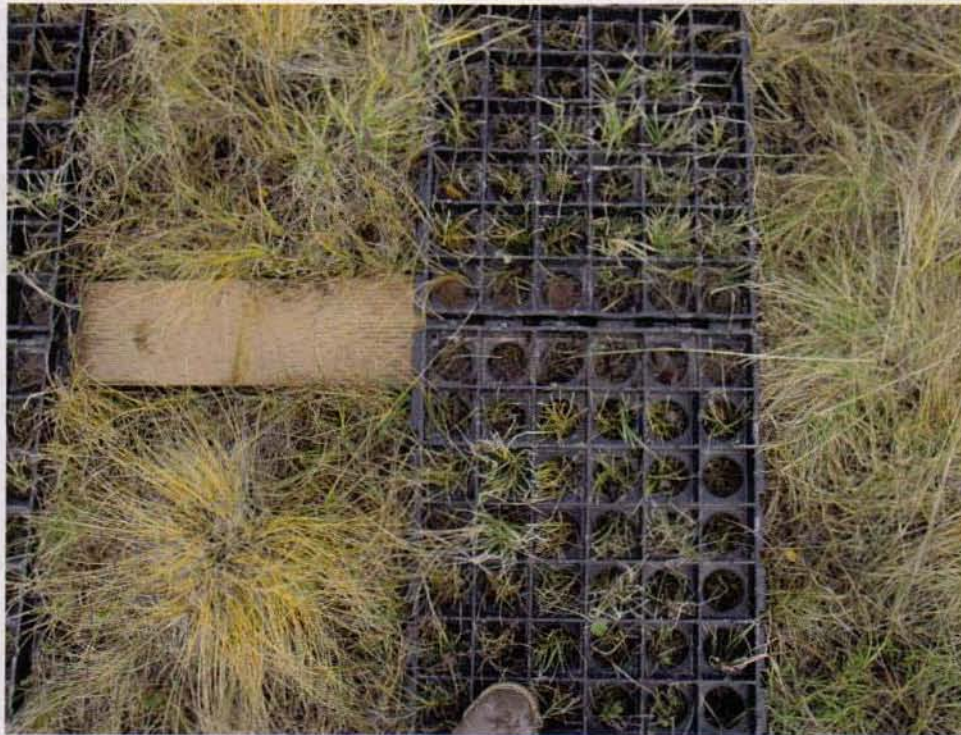
Photo 4. Detail of the cross tie joint. Note 1 5/8" deck screws fastened through the tab edge joints into the underlaying 2X6 cross tie.
