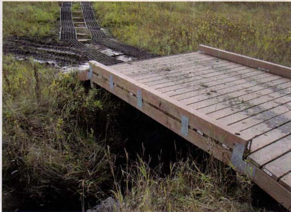
Photo 7. Typical bridge. Four 4X8s are used as underlaying stringers. These are decked with pressure treated 2X6s. Additional 4X8s are used as curb railk. Short 2-3 foot ramps are also constructed out of 4X8s and 2X6 decking. The structure is supported by concrete pilings and additional 4X8 timbers.
