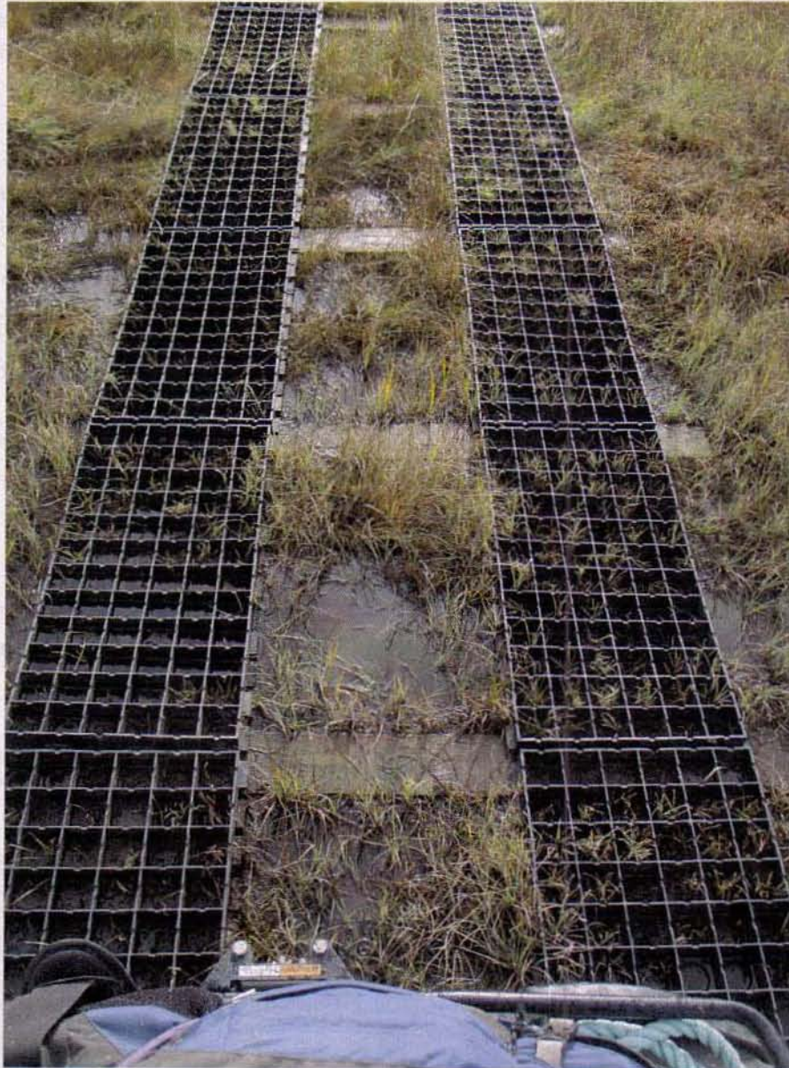
Photo 3. Closeup detail of the GeoTrack configuration. Note cross tie location at 1 meter interval to match length of GeoBlock panels. Note also, the 6 inch inset of the panels on the 6 foot long cross ties resulting in a 5 foot wide tread. At this site little grubbing was required to embed the cross ties. That may not be the case at other locations so labor costs could increase.
