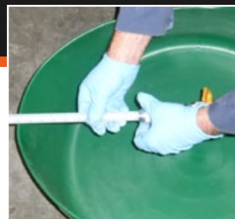
Remove static mixer and dispose of it
