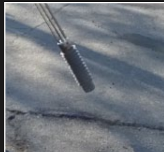
2. Dry pavement with propane torch or heat lance
