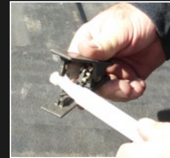
13. Cut static mixer tip
