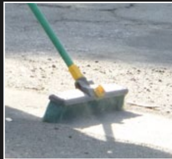
1. Clean pavement with broom or blower
